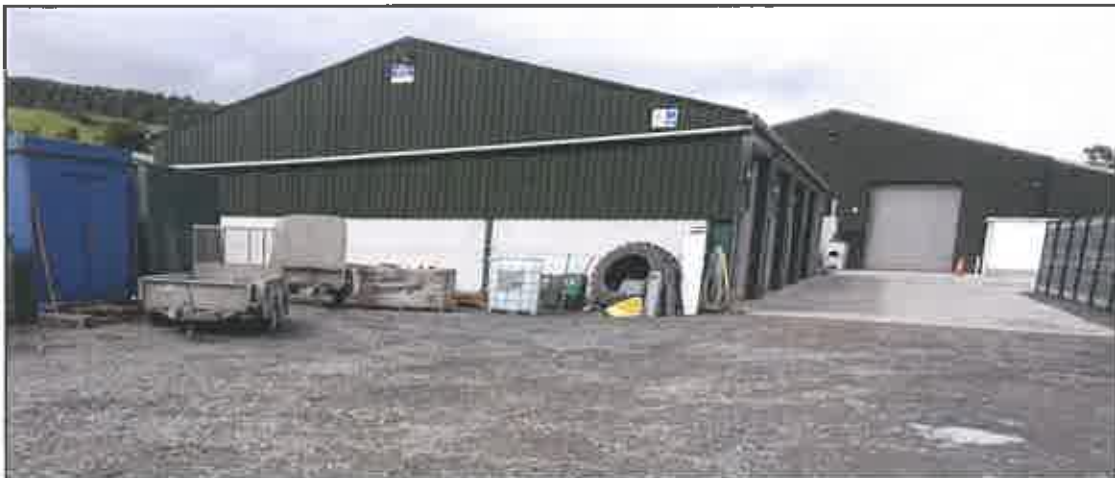
Figure 18: The existing shed south gable. Design and materials are to be the same
